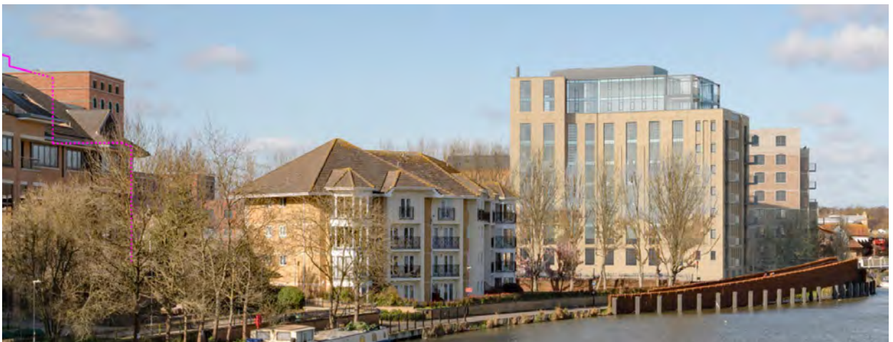
Figure 34 - Zoomed in extract of the winter view P6 from Reading Bridge, with Block D (foreground right), Block E (background far right) and the upper most floors of Block B (background left) – as existing (top), as approved (middle), as now proposed (bottom). Full versions are within Appendix 1.
